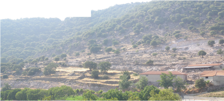
Fig. 4. Area with instability phenomena in tuffs and extremely weathered andesites.
