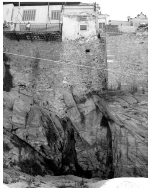
Fig. 3: Location P4. An intensively fractured zone caused by a fault. The wave erosion caused intensive underexcavation to the slope.
