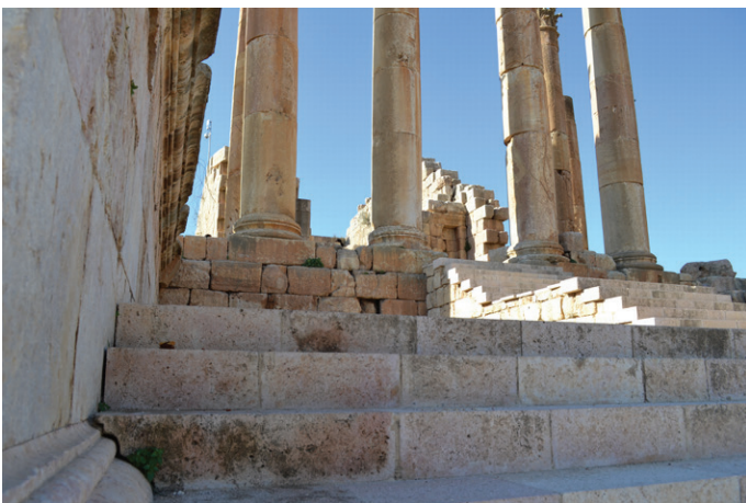
Figure 9: Stone columns on stone foundation, Jerash, Jordan. Photo: D. Gheorghiu
