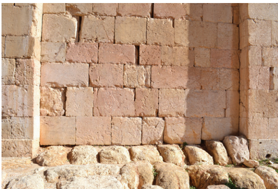
Figure 4: Building foundation, Petra, Jordan. Photo: D. Gheorghiu
