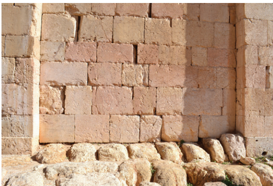
Figure 4: Building foundation, Petra, Jordan. Photo: D. Gheorghiu
