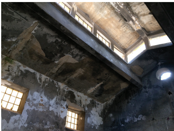
Fig.5 Interior of the second building
