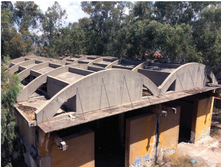
Fig.6 Bird's eyes view of the second building
