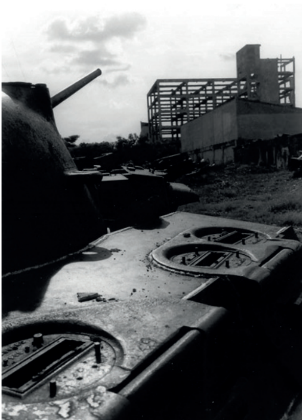
Before: Central Managua, Nicaragua 1994. 35mm photograph, Olympus OM-1 camera, silver gelatine print, 10 X 8 inches, (Intencity AFP 2004). Building destroyed by 1972 Earthquake with derelict armoured vehicle from 1979 revolution. Author.
