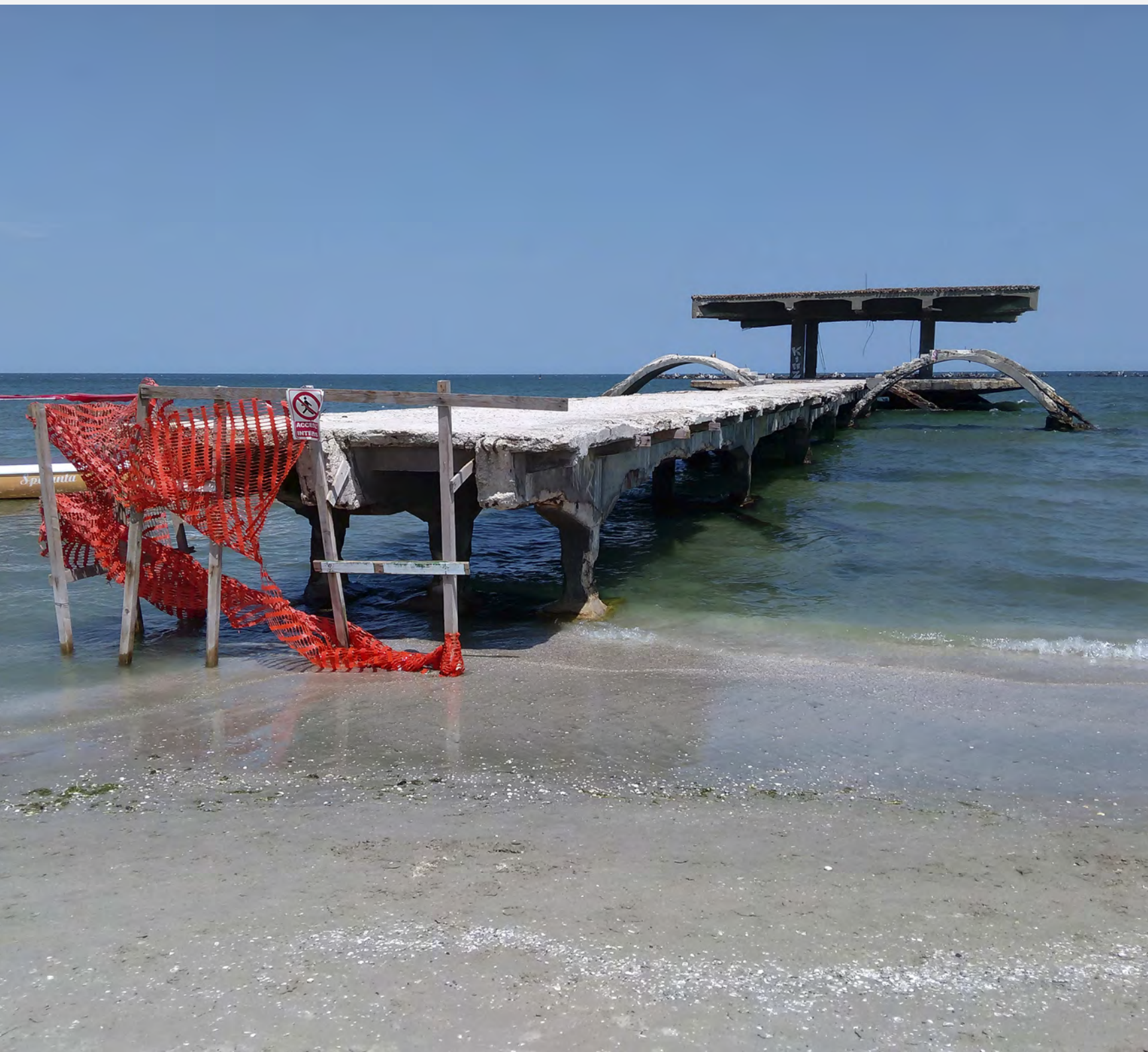
Figure 7. Former beach, Ola harbour in Mamaia, 2015
