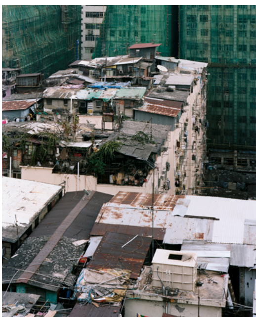
Figure 12: Building 5, Tai Kok Tsui Area
