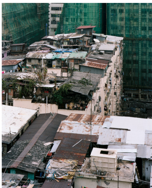
Figure 12: Building 5, Tai Kok Tsui Area
