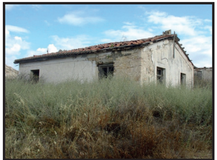
Figure 9: Building 3, as seen from the coastal road D1. Photo: M. Delazanou (2020)
