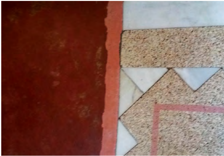
Figure 6. T. Marthas: Interior floor detail of the T. Marthas' residence-atelier in Kalamaki, Athens. Source: Archive of Takis Marthas.
