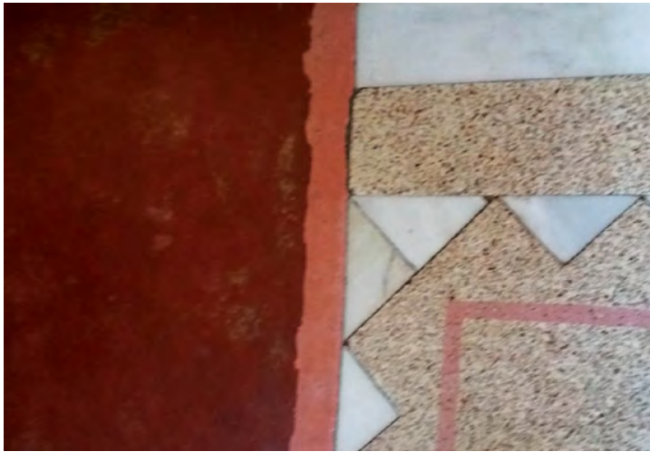
Figure 6. T. Marthas: Interior floor detail of the T. Marthas' residence-atelier in Kalamaki, Athens. Source: Archive of Takis Marthas.
