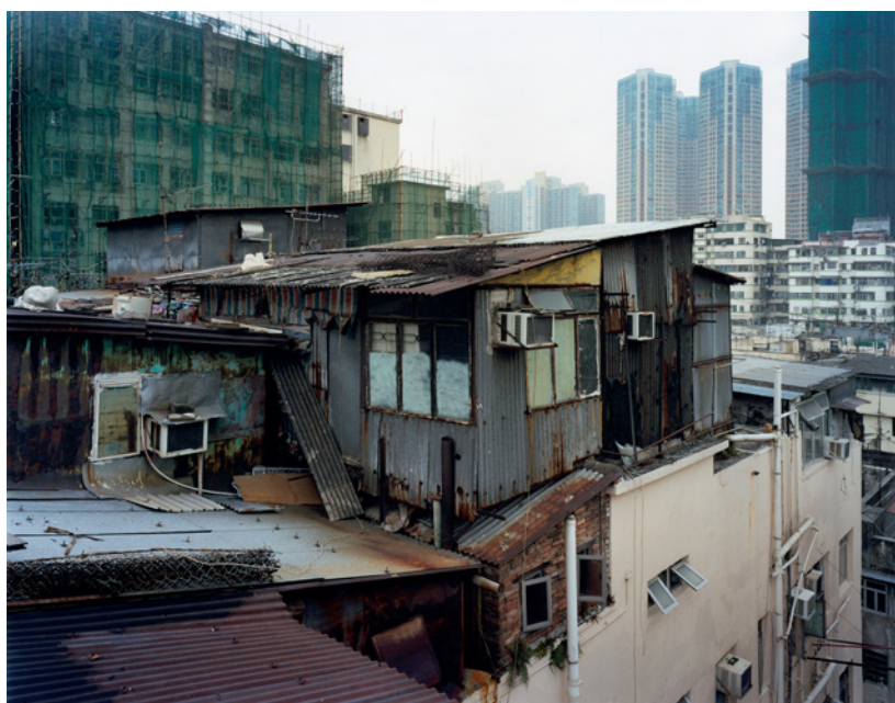
Figure 13: Building 5, Tai Kok Tsui Area
