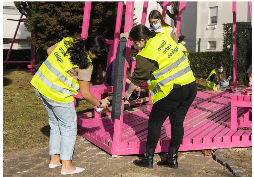
Figure 2. Students working on one of the five wood structures built, Matosinhos, Portugal, December 11, 2021. (Source: ESAD Archive, Fernando Miranda, December 11, 2021.)
