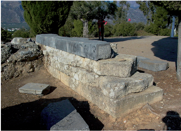
Fig. 2. The foundations and crepis of the Throne in situ (photo: G. Alevras).
