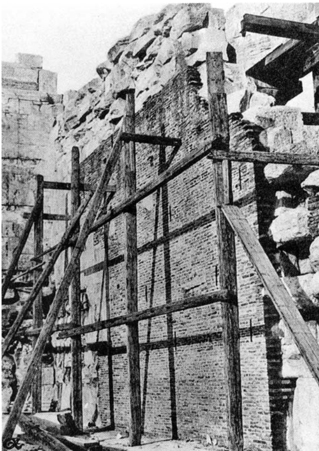
Fig. 3. Restoration and reconstruction works on the Acropolis ca. 1840 (photo: N. Balanos).
