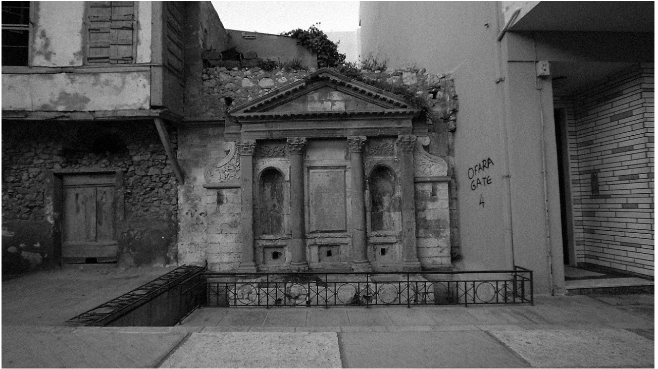
Fig. 12. Herakleion, Priuli Fountain, 1666 (photo: author).
