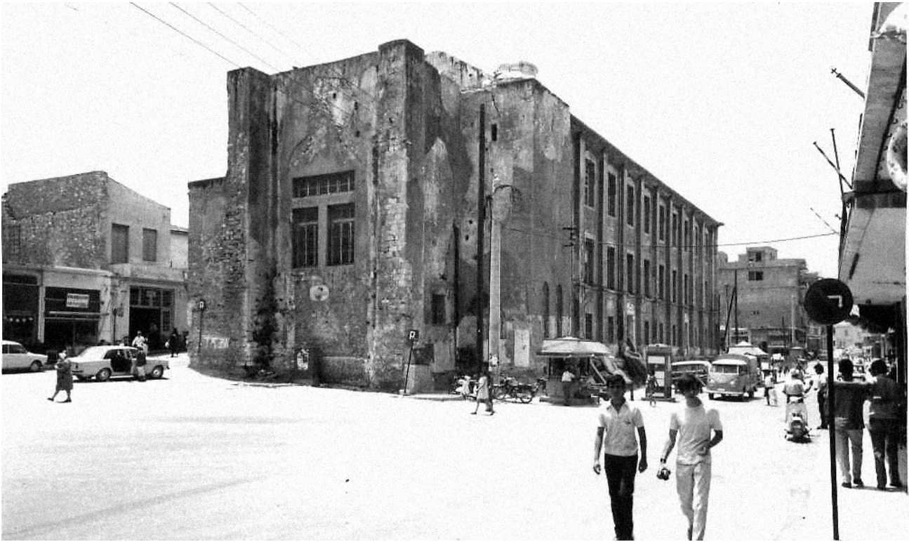
Fig. 3. Herakleion, San Salvatore before demolition, 1972.
