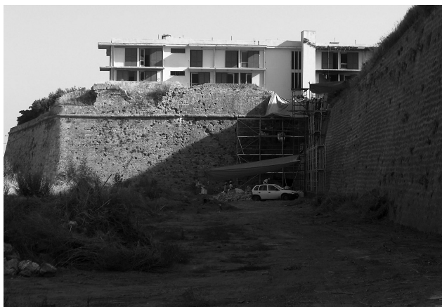
Fig. 11. Chania, Hotel Xenia on the seafront bastion of the Venetian wall. Before demolition, 2007.
