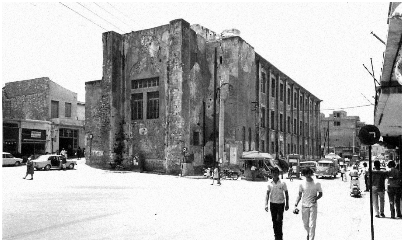
Fig. 3. Herakleion, San Salvatore before demolition, 1972.
