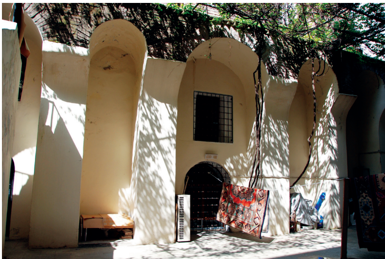
18. Terrace of the Myrelaion church (after 920), view from the south, photo: Piotr L. Grotowski.
