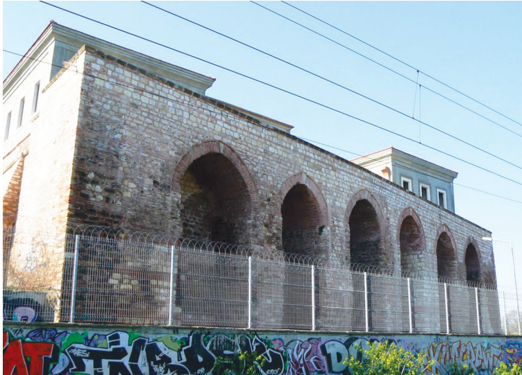
15. Terrace of the Gülhane Hospital, view from the east, photo C. Cangul.
