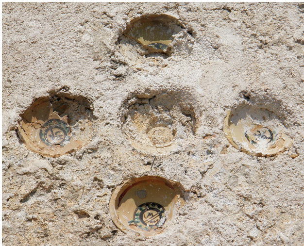
Figure 26: Bacini assemblage consisting of bowls of the polychrome glazed pottery (“RMR Ware”), immured in Agios Antonios, in Angeliana (Rethymnon, Crete) (photo: by the author).
