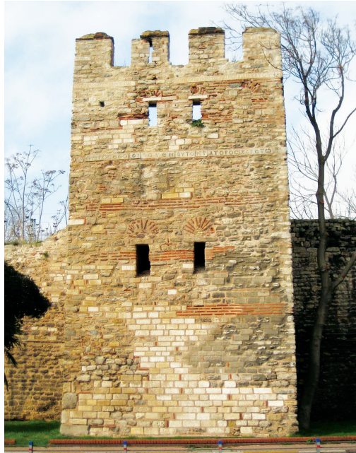
9. Theophilos' tower heightened by Leo VI in 906, elevation from the sea side (east), photo: Piotr L. Grotowski.
