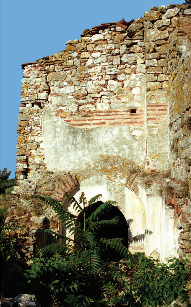
Fig. 6. Apollonia Lake. Monastery of St. Constantine. Katholikon. View of the northwest corner bay from the west.
