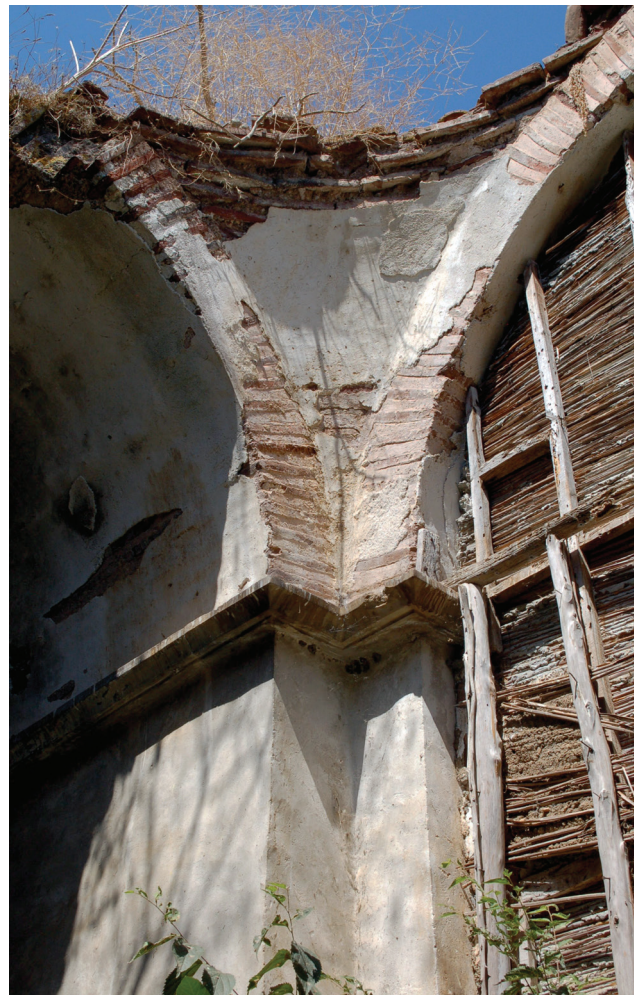
Fig. 17. Apollonia Lake. Monastery of St. Constantine. Katholikon. Interior view towards the northwest.
