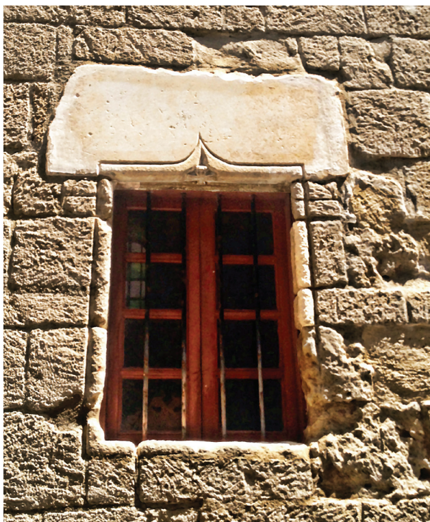
Fig. 13. Telos, katholikon of Hagios Panteleemon, South façade. The marble lintel of the window.
