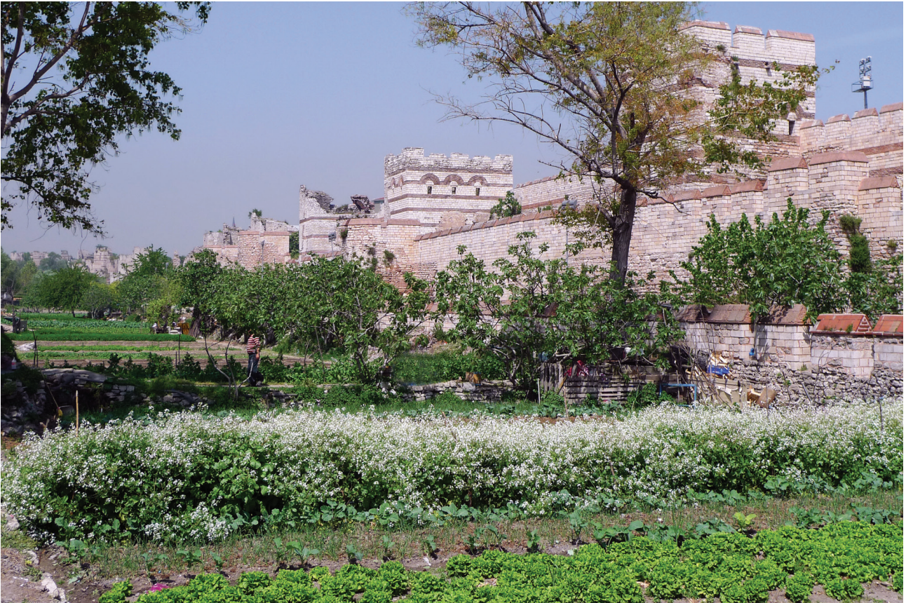
Fig. 1. Constantinople. The land walls seen from south-west with the ditch, outer wall and inner wall, tower 25 in the foreground.
