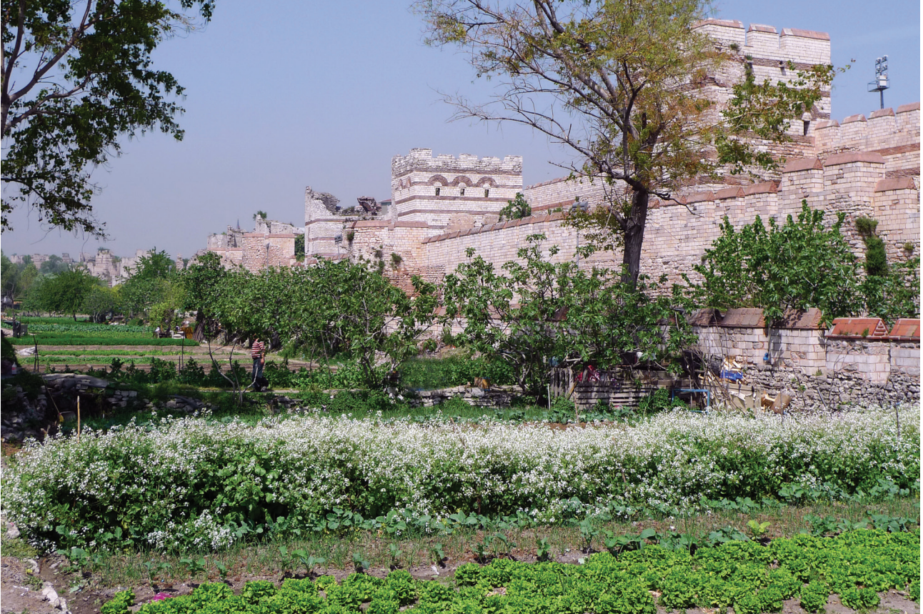
Fig. 1. Constantinople. The land walls seen from south-west with the ditch, outer wall and inner wall, tower 25 in the foreground.
