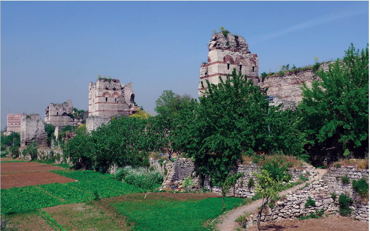
Fig. 6. Constantinople. Towers 18-22 in the inner circuit, outer wall and ditch seen from south-west.
