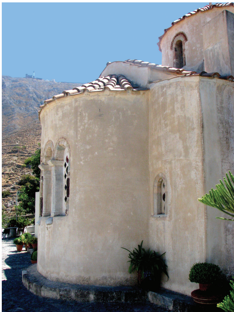
Fig. 10. Santorini. Episkopi in Mesa Gonia. Northeast view.
