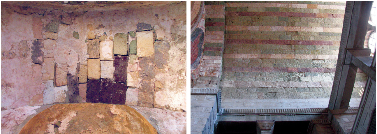
Fig. 3. (a) Naxos. Hagios Mamas near Potamia. Barrel vault. (b) Paros. Katapoliani. Main church. Barrel vault.
