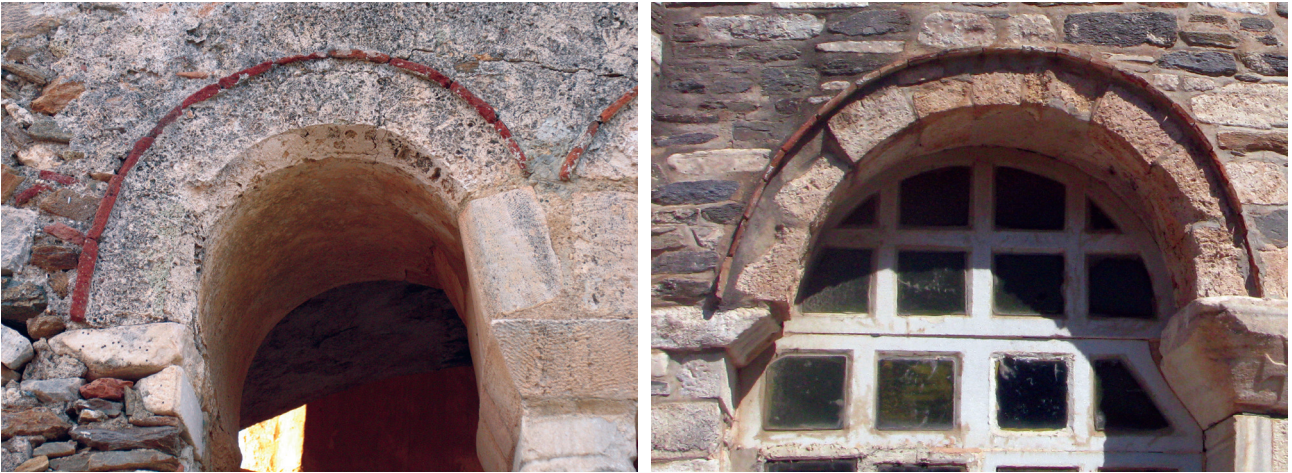
Fig. 2. (a) Naxos. Hagios Mamas near Potamia. South window arch. (b) Paros. Katapoliani. Main church. Apse window arch.
