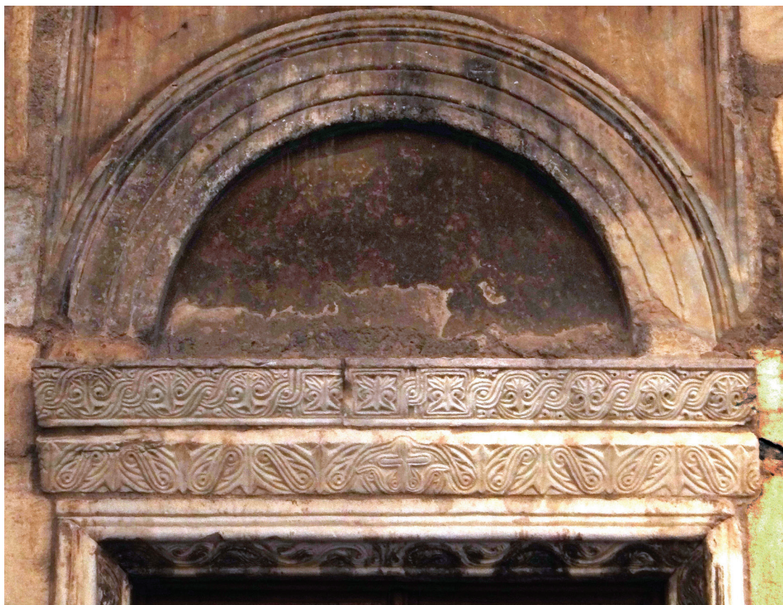
Fig. 9. Athens, The church of the Panagia Gorgoepekoos. Spolia as lintel of the north entrance.
