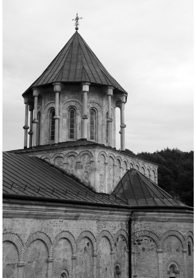
Fig. 7. Serbia, monastery of Hopovo, church of St. Nicholas. The dome and part of the south facade.
