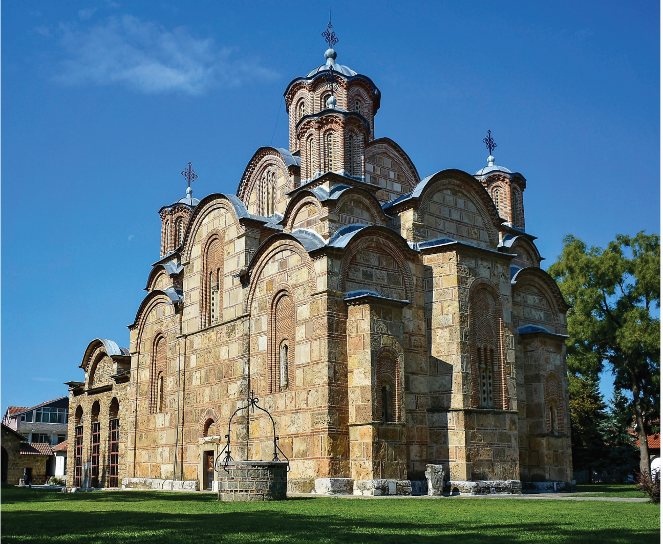
Fig. 1. Gračanica, church of the Dormition of the Virgin. View from northeast.
