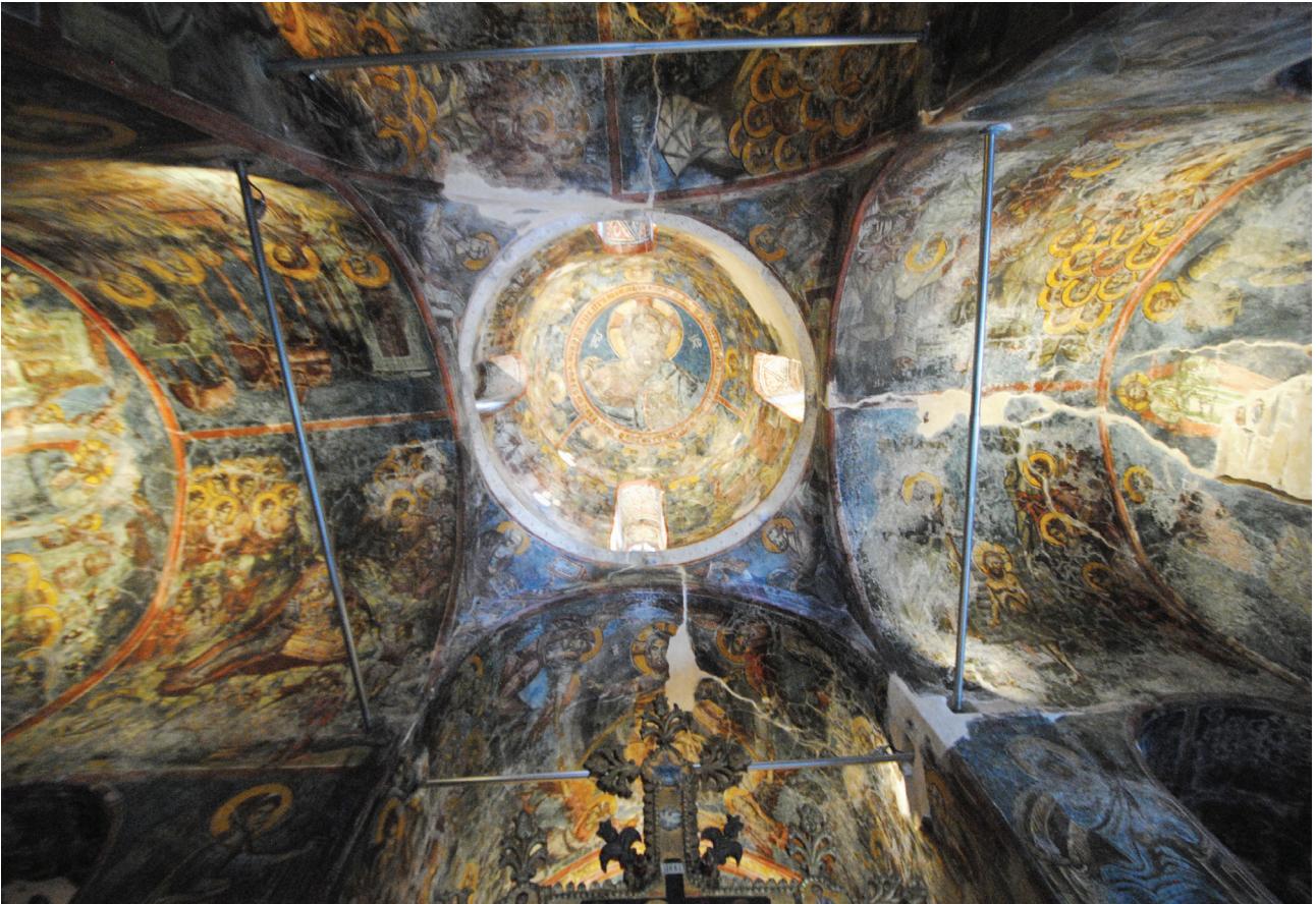
Fig. 18. Kastania (Mani), Hagios Petros. View into vaulting.
