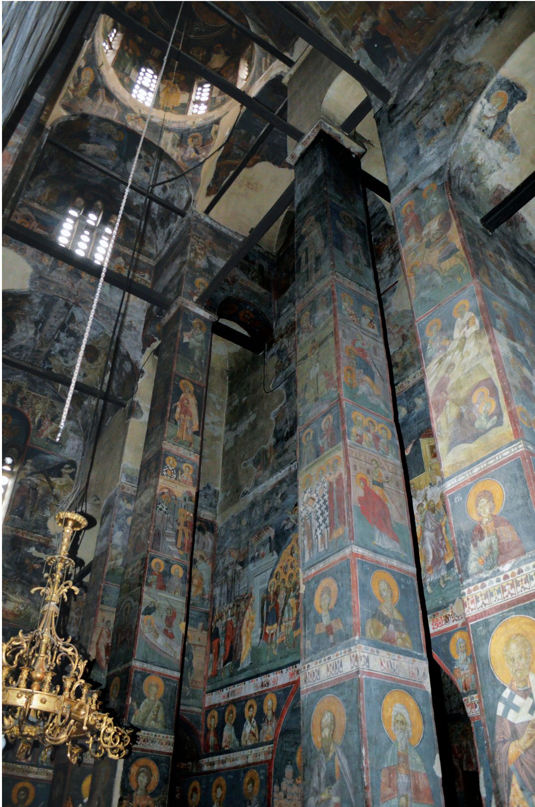
Fig. 2. Gračanica, church of the Dormition of the Virgin. View into the naos vaulting.
