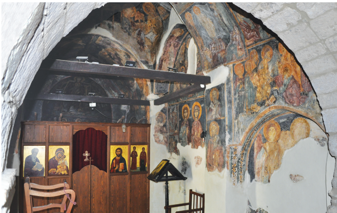
Fig. 4. Naos. South wall, view from Northwest.
