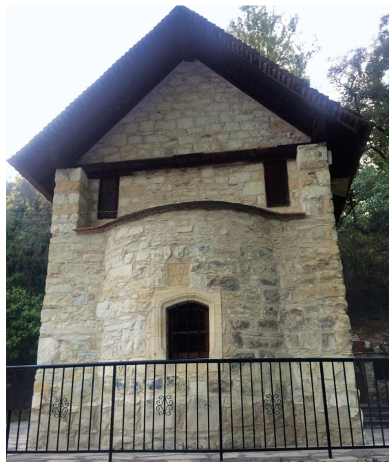
Fig. 1. Limassol, Koilani, the church of Saint Mavra. View from East.
