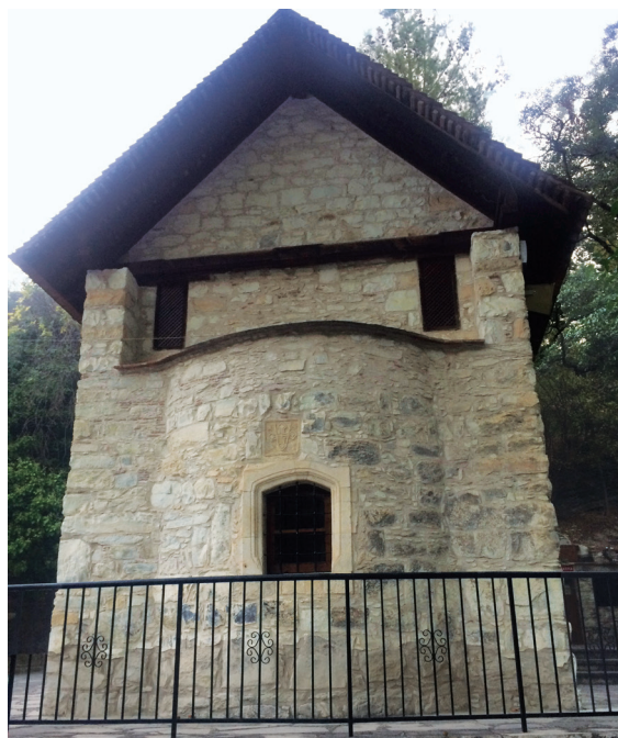
Fig. 1. Limassol, Koilani, the church of Saint Mavra. View from East.
