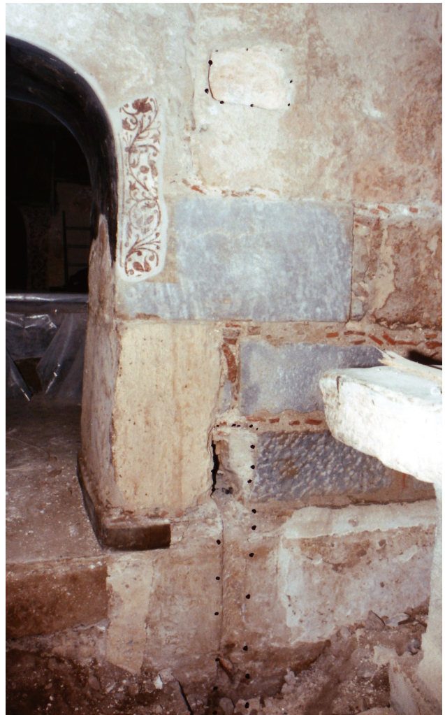
Fig. 7. Panagia Skripou. Grooves cut on the side walls of Saint Peter's chapel to attach the marble screen.
