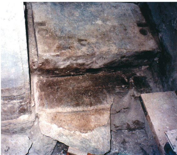
Fig. 6. Panagia Skripou. Narthex, south door. (a) The remaining timber tie-beam and the frescoes covering the walls. (b) The threshold of the south door with parts of the original marble floor.
