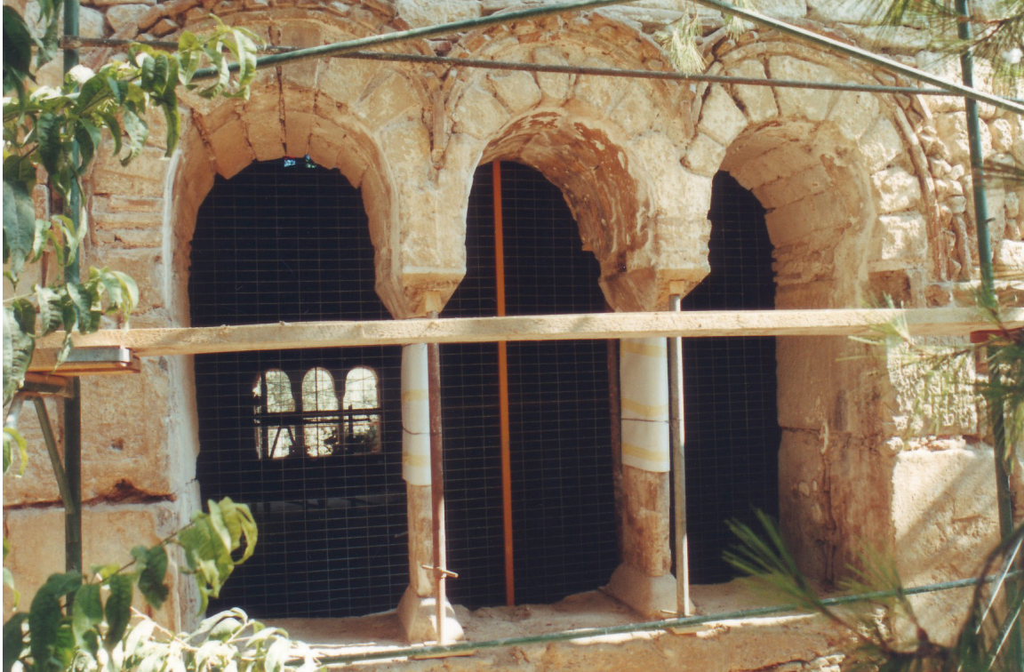
Fig. 2. Panagia Skripou. View of the south transept window after works.
