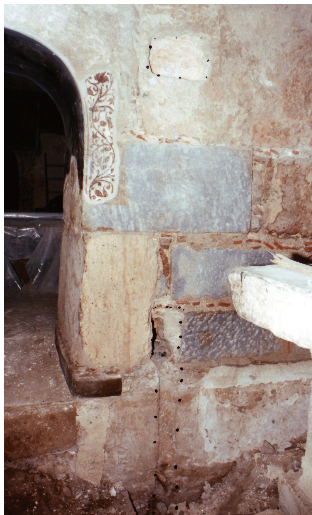
Fig. 7. Panagia Skripou. Grooves cut on the side walls of Saint Peter's chapel to attach the marble screen.
