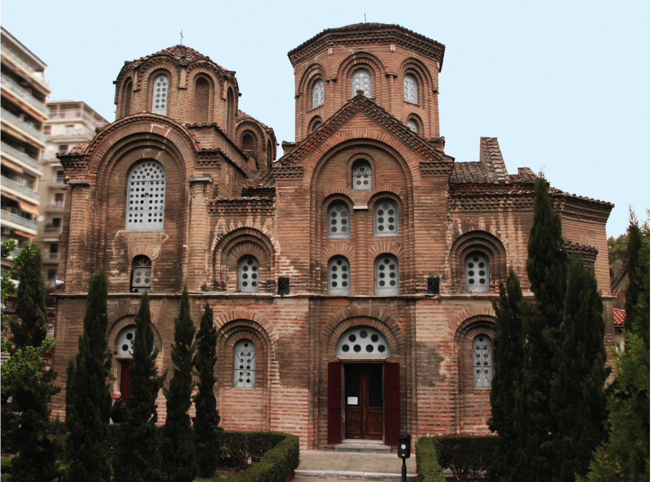
Fig. 7. Thessaloniki, Panagia Chalkeon, 1028. View from the South.
