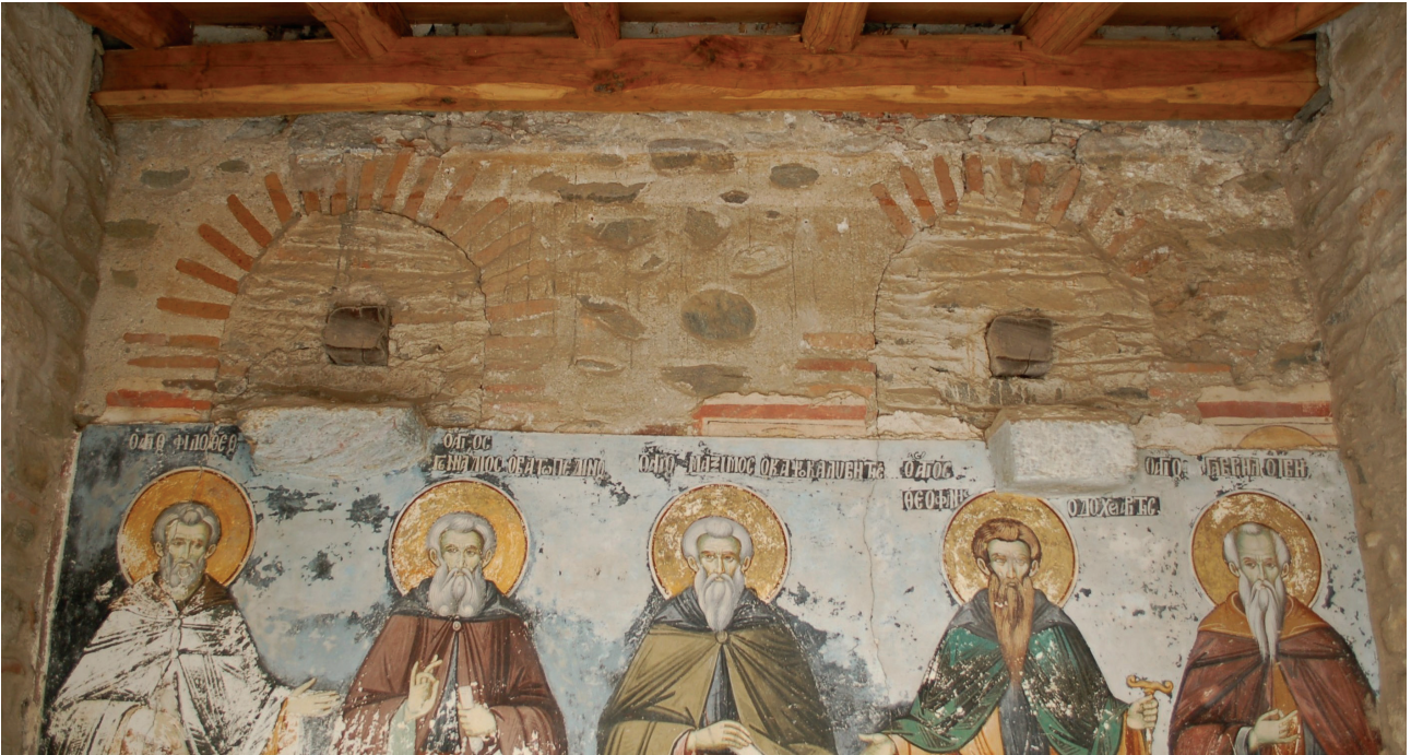
Fig. 6. Karyes, Protaton church. Detail of the masonry of the north façade (March 2011).
