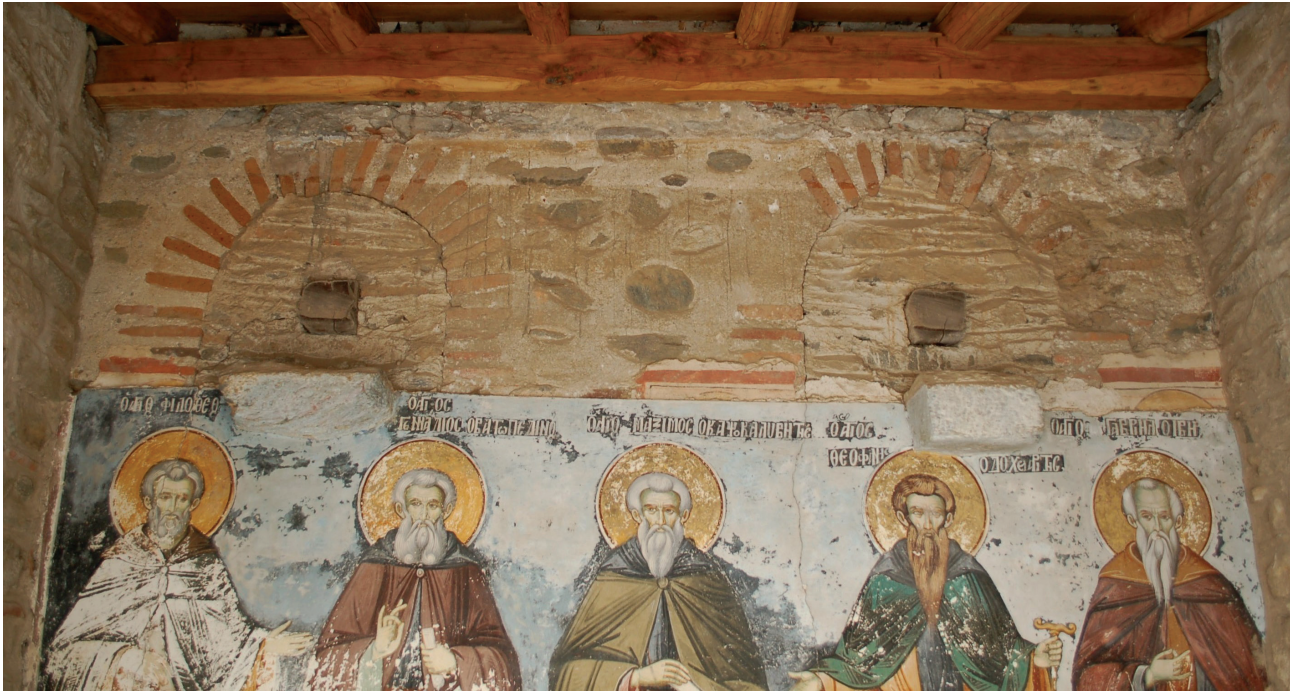
Fig. 6. Karyes, Protaton church. Detail of the masonry of the north façade (March 2011).
