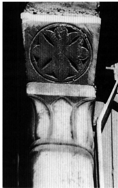
Fig. 13. Impost over a modern mullion on the south façade.
