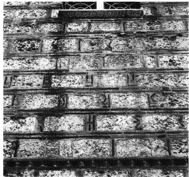
Fig. 15. Detail of the masonry on the south façade.
