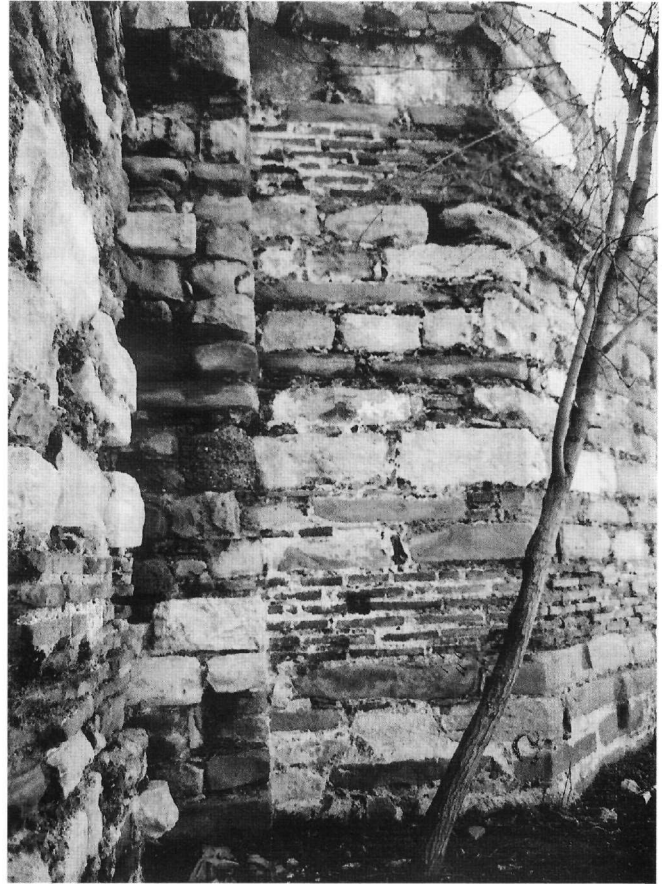
Fig. 10. The brick courses end at the corner where walls 'e' and 'd' of tower II meet.
