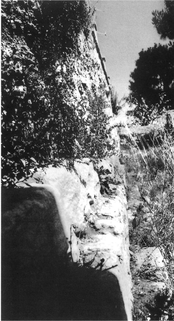
Fig. 3. The wall 'n'.
