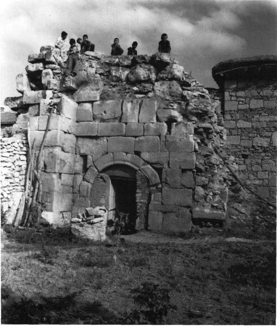
Fig. 7. Yürme, church of St. Michael. Detail of west façade.
