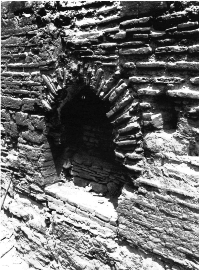
Fig. 9. Istanbul, Christos ho Pantepoptes . South façade, detail of niche.
