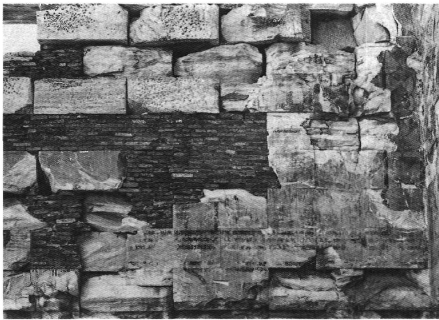
Fig. 9. Chevron and spindle ornament. Parthenon church, south wall, west end (photo: after Collignon, pl. 135A).
