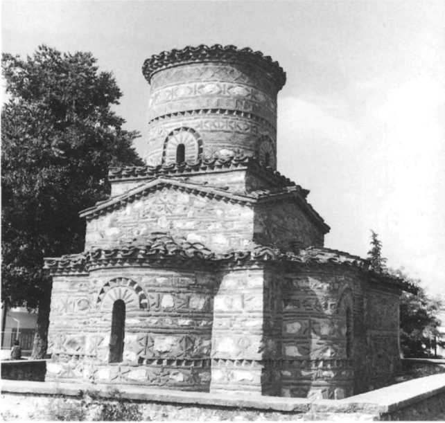
Fig. 3. Kastoria, Panagia Kubelidike. From the northeast.
