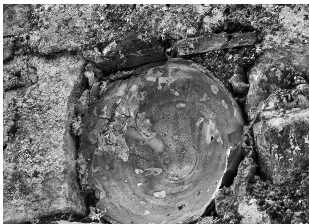
Fig. 2. Neftis-Amari, church of Sts Theodoroi. Detail showing the way the vessel is immured in the wall.
