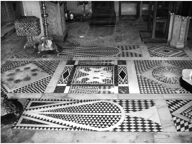
Fig. 2. Mega Spelaion, katholikon. View of the central part of the pavement from the north. It is noted that this area has been restored, but the original design has been reproduced accurately, as the form of the pavement is identical in the picture published by Soteriou in 1918 (see n. 1), where the original parts were still extant.
