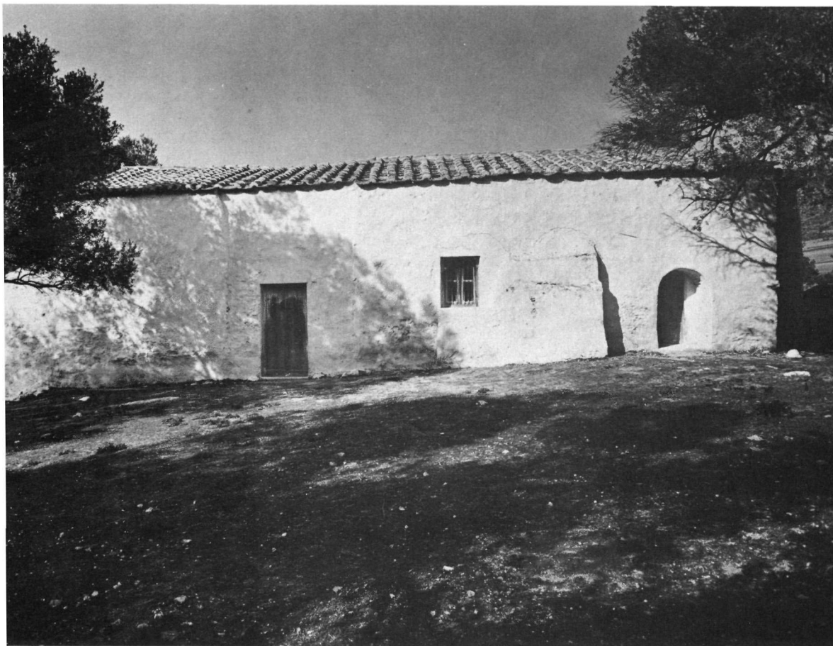
St. George at Kouvaras. View from the South.
