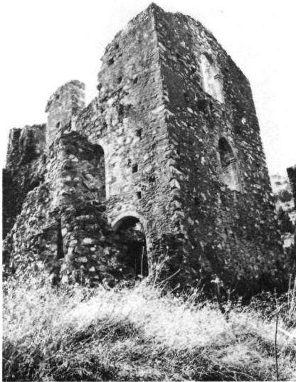
Fig. 12. Mistra. Late Byzantine house north of the palace. View from the Northeast.
