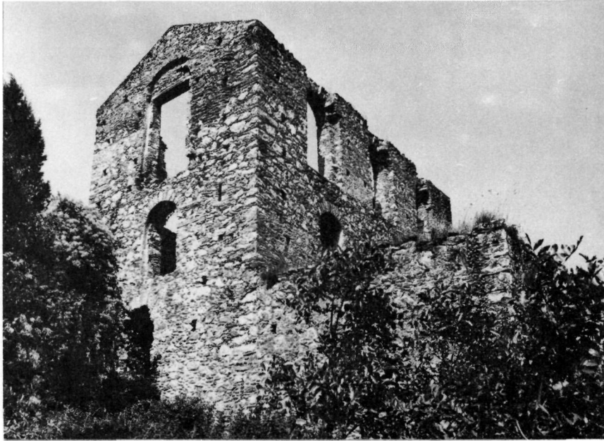
Fig. 14. Mistra. The late Byzantine «House Γ». View from the East.
