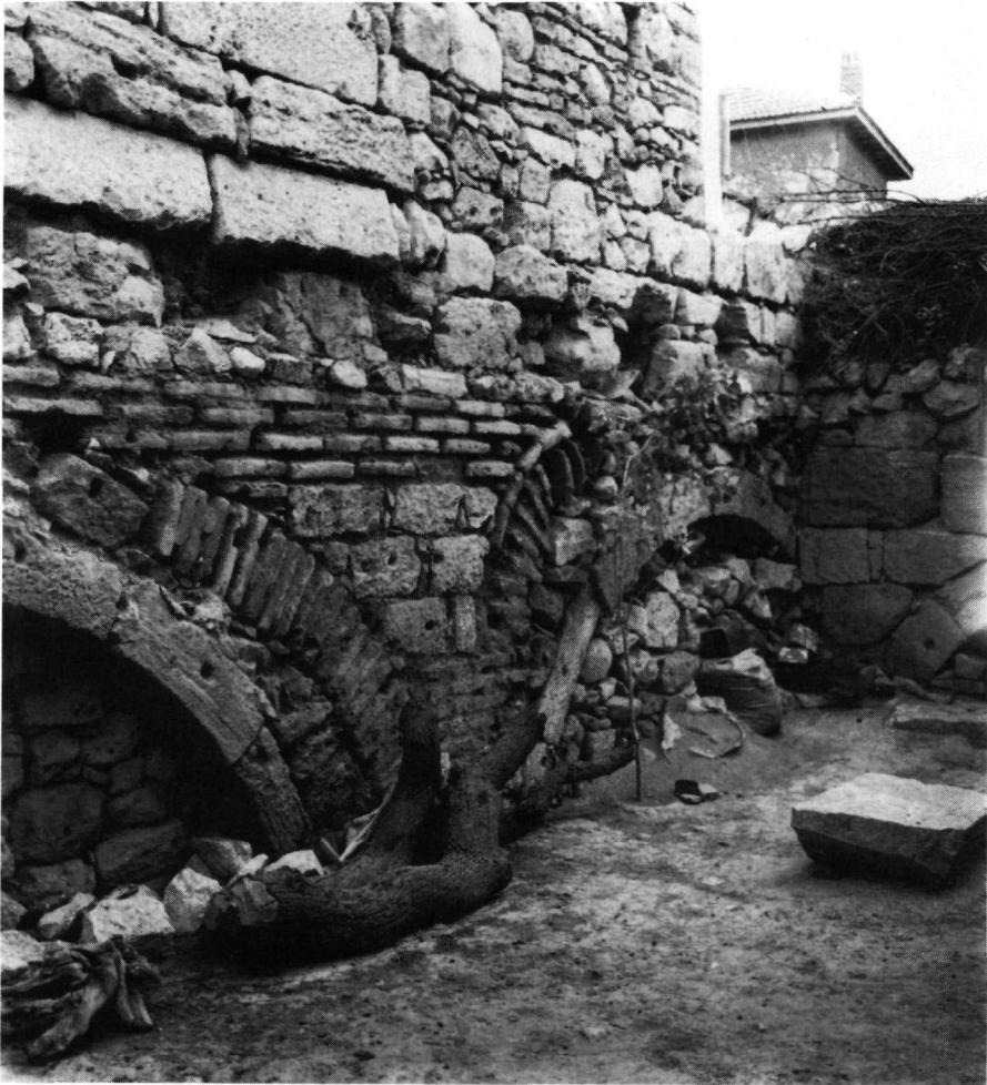
Fig. 8. Yürme, church of St. Michael. North crossing, showing two structural phases.
