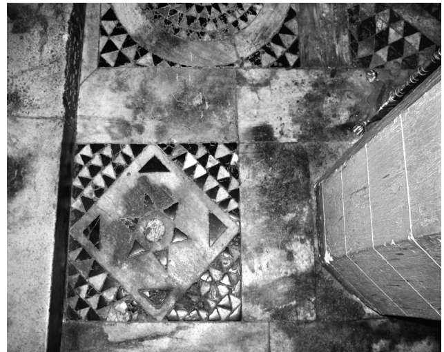
Fig. 11. Mega Spelaion, katholikon. A star incrustation on a marble slab. The relation of the pavement to the pier is noted.
