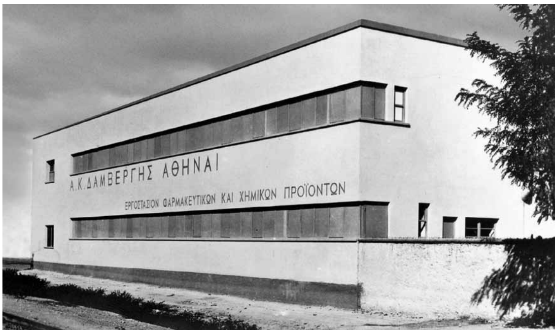
Figure 5. The factory of the Damvergis Pharmaceutical Company, established in 1932.
