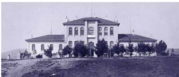
Figure 9. The building of the Pendik Veterinary Control Institute at the time of establishment. https://vetkontrol.tarimorman.gov.tr/pendik/Sayfalar/Detay.aspx?SayfaId=45
