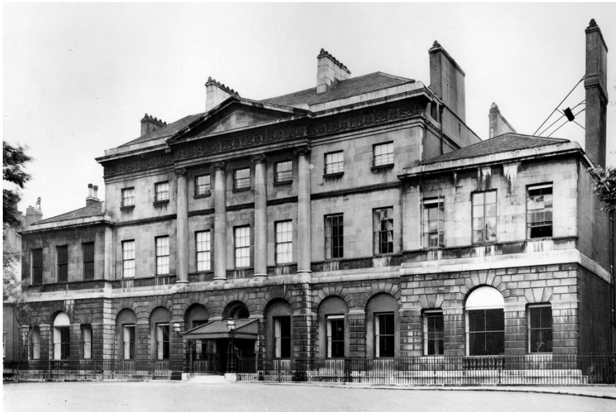
Fig. 1. Lansdowne House, Façade
