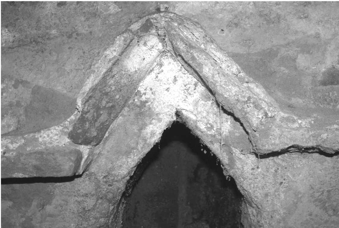
Fig. 19 The arched spring with the band of red tiles and the layer of plaster over it.
