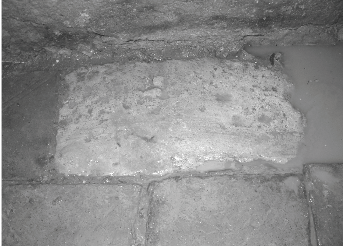
Fig. 12 The Fountain House the limestone floor slab.
