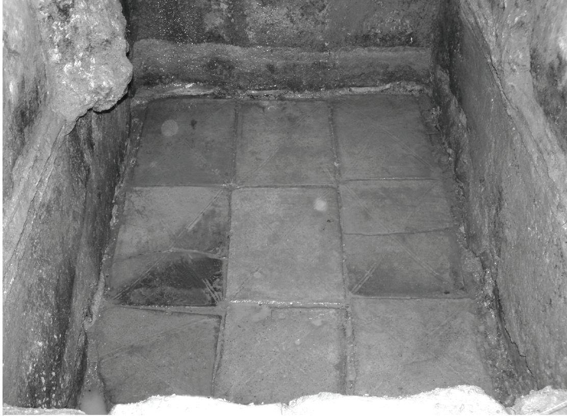
Fig. 10 The Fountain House: the floor with tiles and the natural rock projections below the large tunnels.
