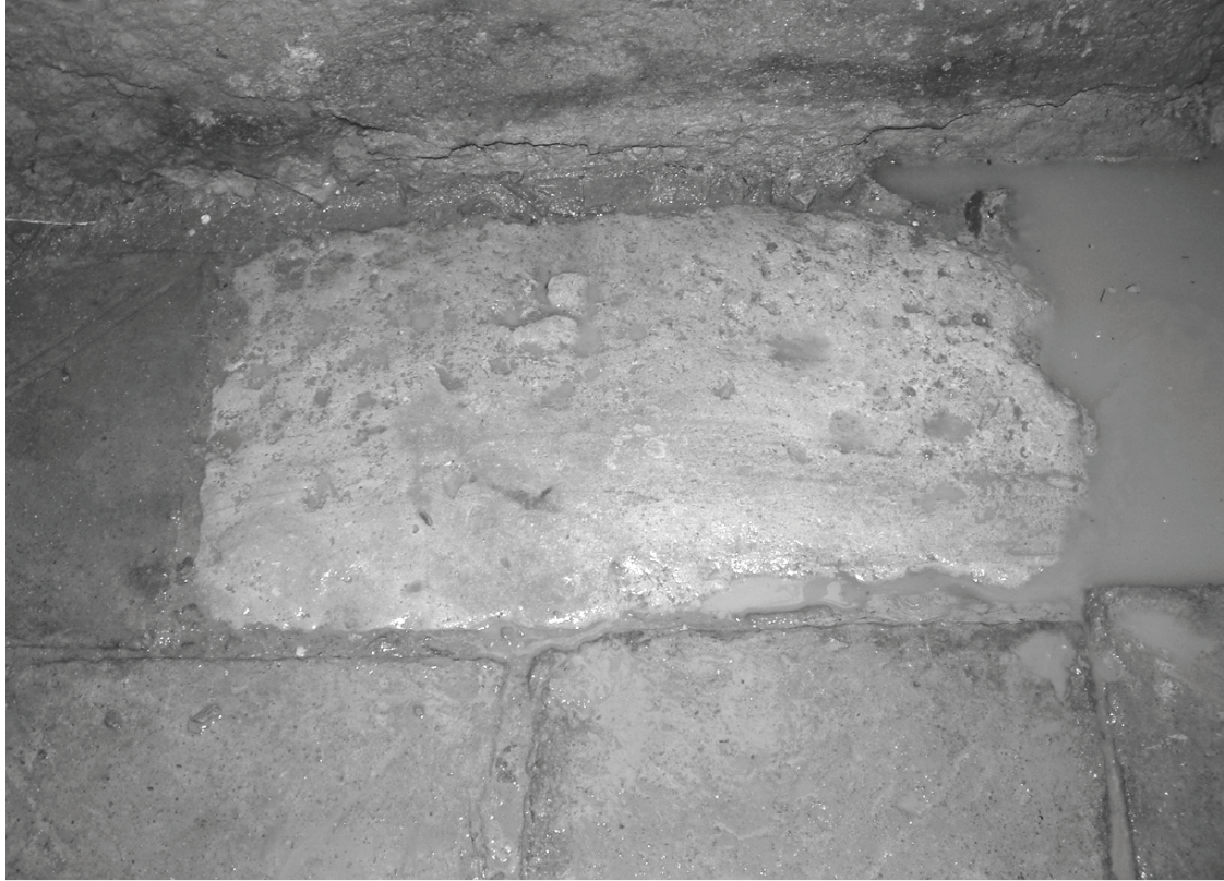
Fig. 12 The Fountain House the limestone floor slab.
