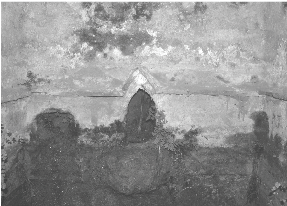
Fig. 13 The two springs: the one defined by the arch discharges into a channel that runs along the natural rock projection.
