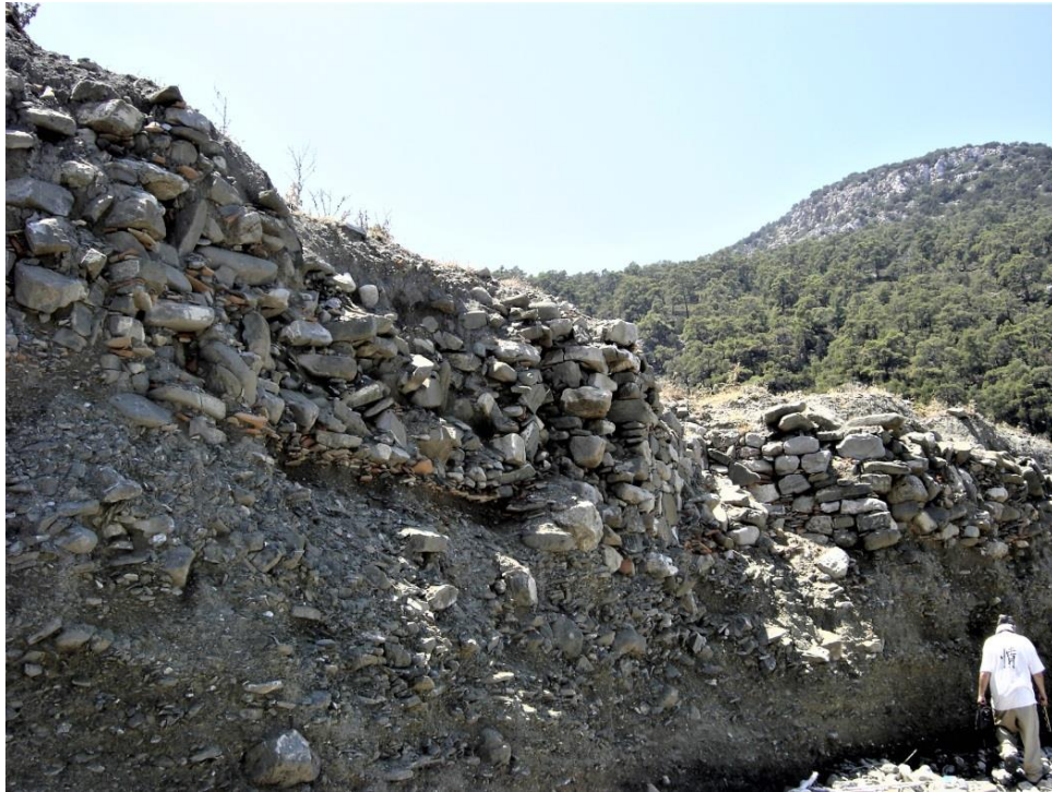
Figure 13. Site Glyphada. Remains of collapsed constructions by the shoreline (Source: KARP).
