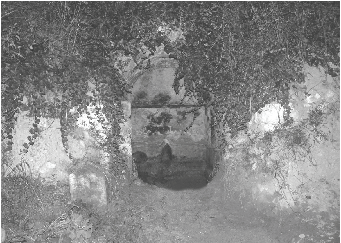
Fig. 4 The Fountain House from east.
