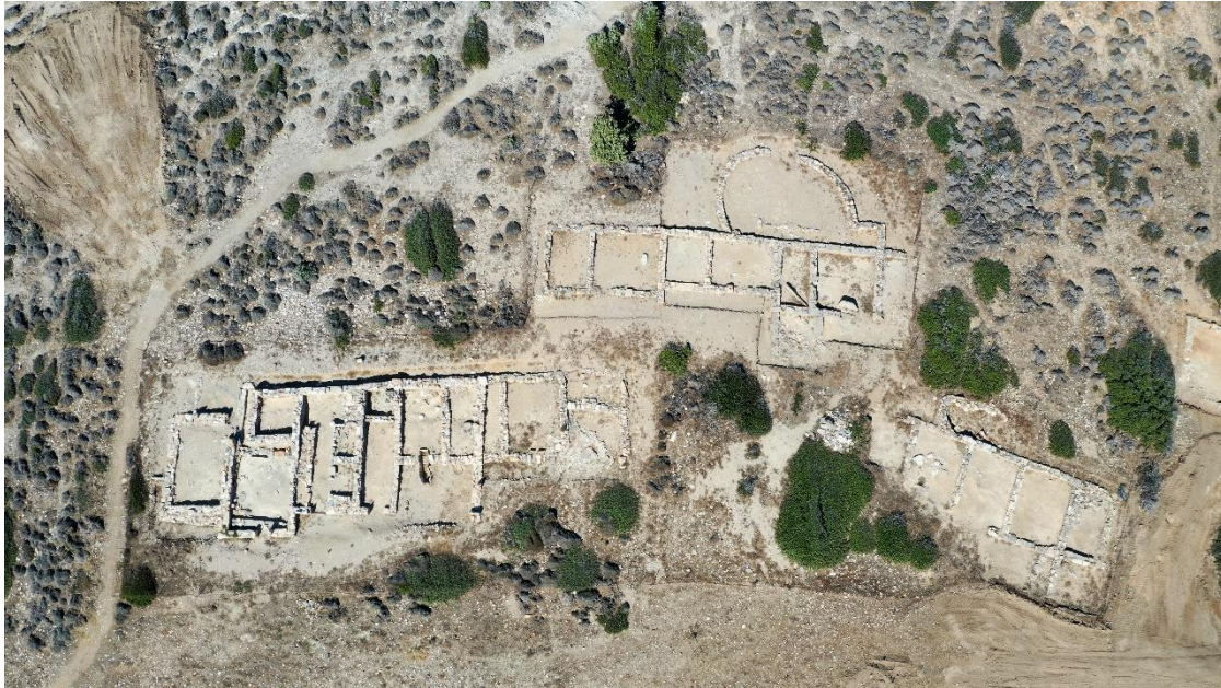
Fig. 6. Aerial photo of Buildings B, H, P (courtesy Y. Kourayos).
