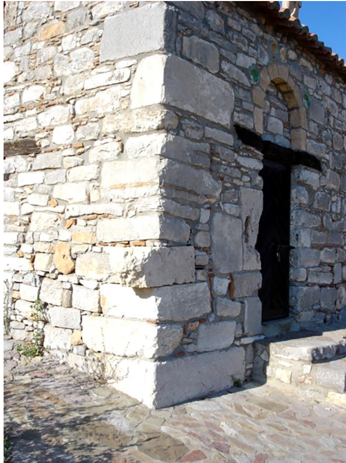
Figure 19. Monolithos village. St Thomas' church with reused ancient material (Source: KARP).
