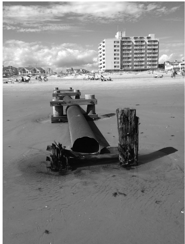
4. Typical resort development in cohabitation with obsolete sewage overflow tubes that helped flash to the ocean the excess of water after a storm event. Atlantic sand barrier, Ocean City, New Jersey.
