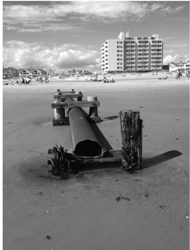
4. Typical resort development in cohabitation with obsolete sewage overflow tubes that helped flash to the ocean the excess of water after a storm event. Atlantic sand barrier, Ocean City, New Jersey.
