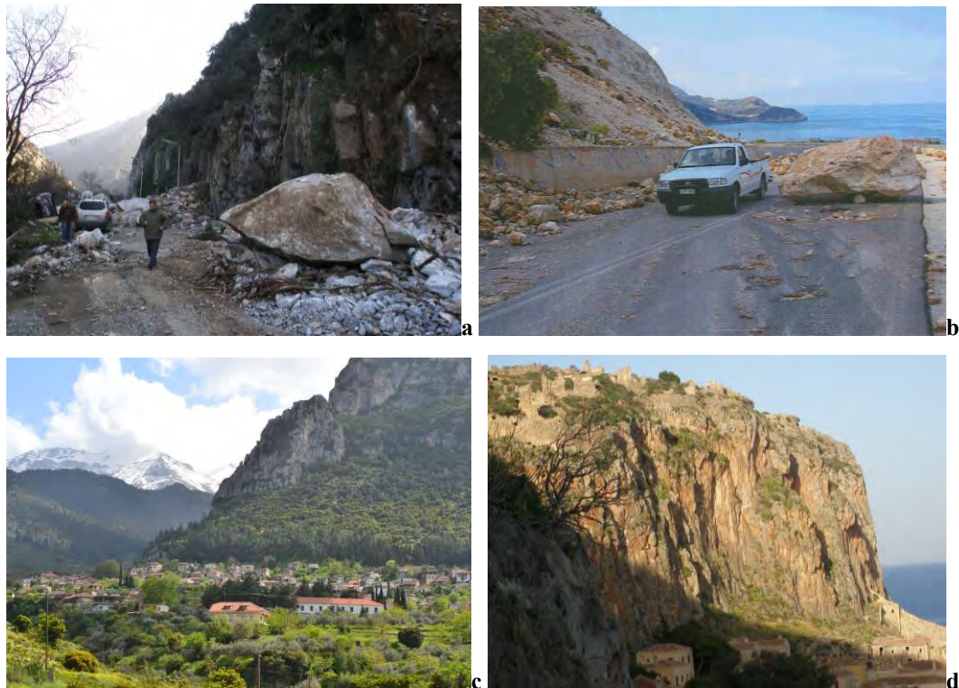
Figure 3 - Impact of rockfall a) on highway in Tempi valley b) on roadway during Lefkada earthquake (photo from Geobruigg), c) Tithorea village, d) Monemvasia archaeological site.
